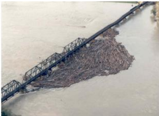
1995 Skagit River Flood – BNSF Bridge failure
